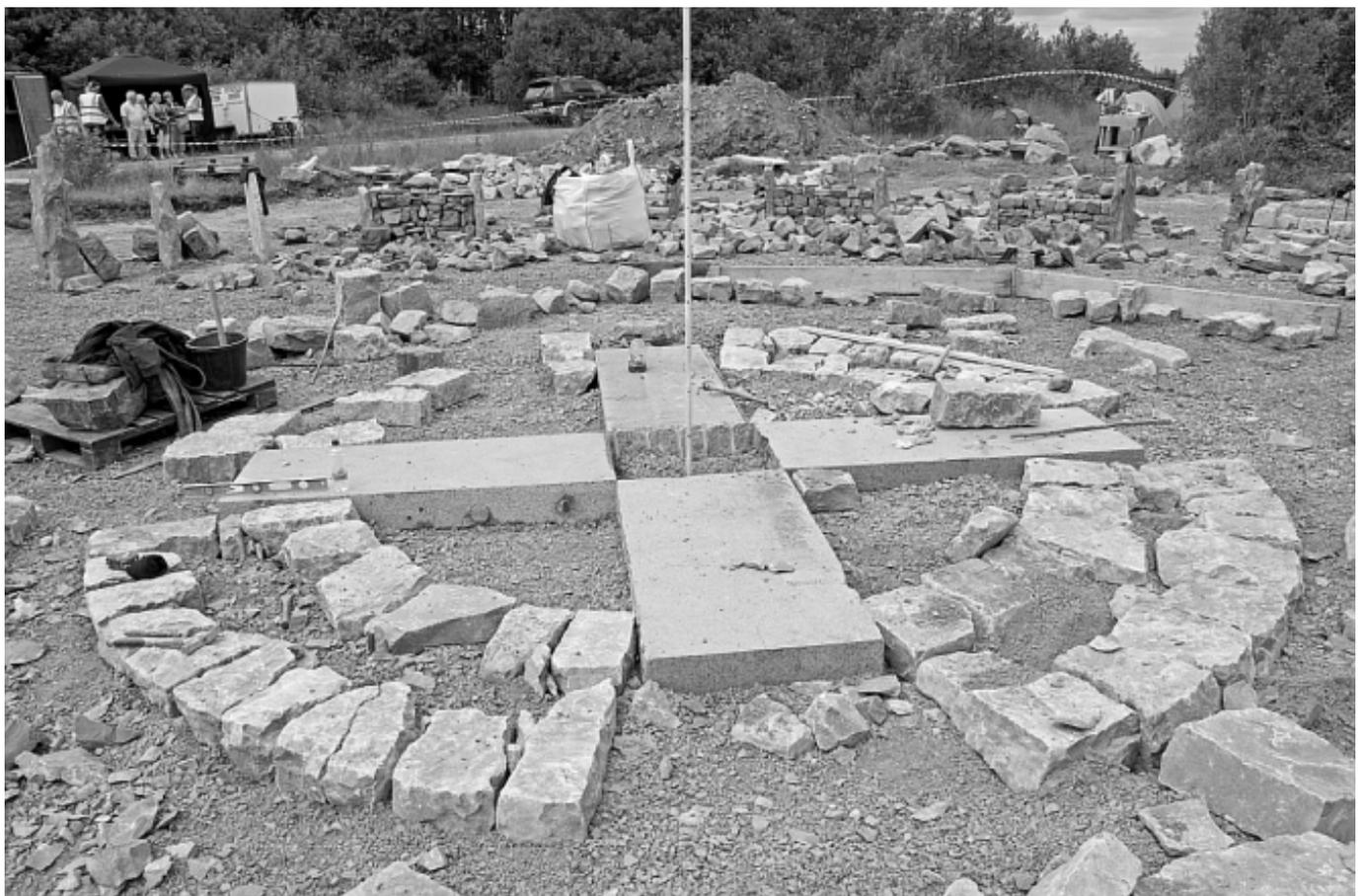
The inner circle has a limestone outer wall (from Co. Roscommon, Connaght), whilst the inside is being built with bands of stone from various areas. Local sandstone forms a lower band, above this is green sandstone (Co. Laois, Leinster), within which niches are being built to take hand carved 600mmx 600mm shields of the provinces, donated and carved by members of the Association. The bands above this will vary in thickness depending on the donated stone.
